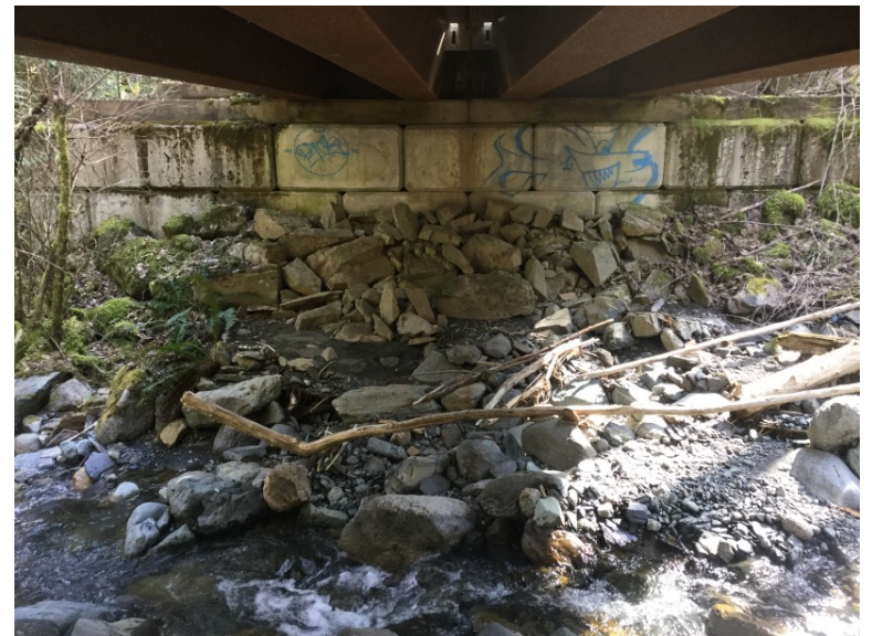
Right Bank Abutment when facing downstream
