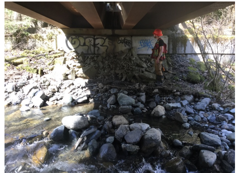
Left Bank Abutment when facing downstream
